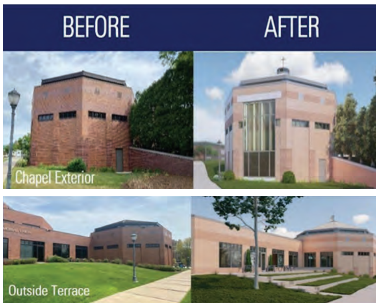
Renovations to outside of Chapel of the Holy Family in Milwaukee Wisconsin.
